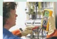
Insulation test at a distribution panel
